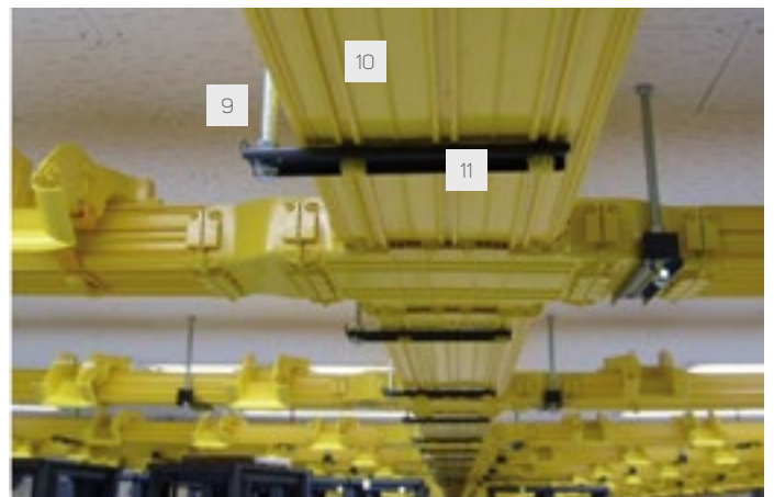
2. OptiWay ceiling installation
