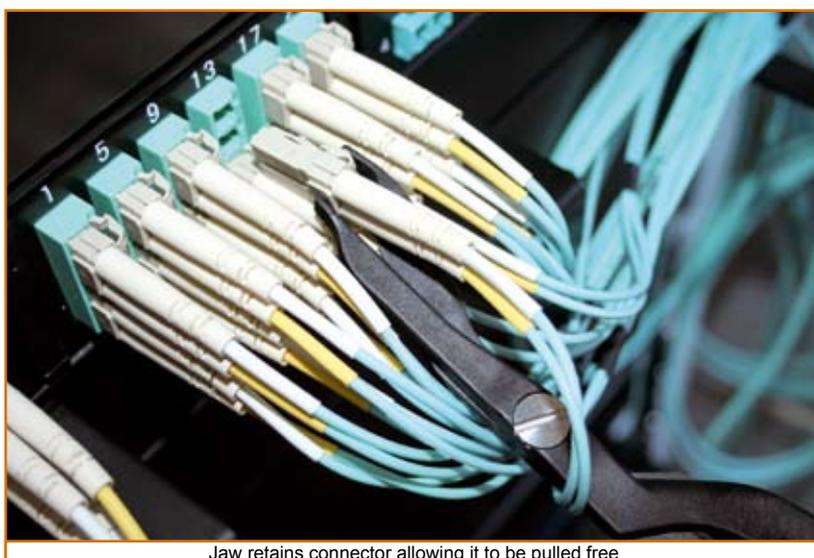
Jaw retains connector allowing it to be pulled free
